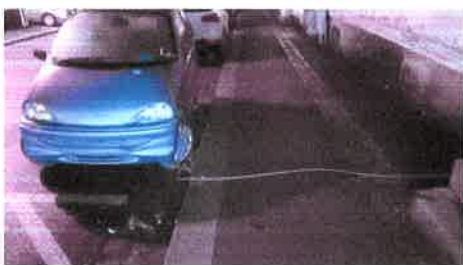
Fig 9– Kabel over fortau - langs vegg - inn vindu
